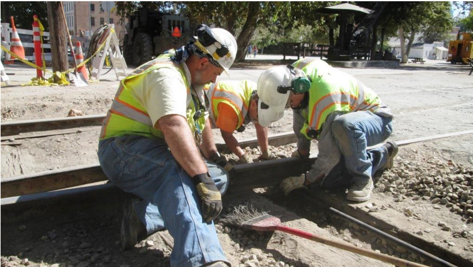
Mike F., Joe, and Steve work at securing the clamps of the gauge-rod onto the base of the rail
