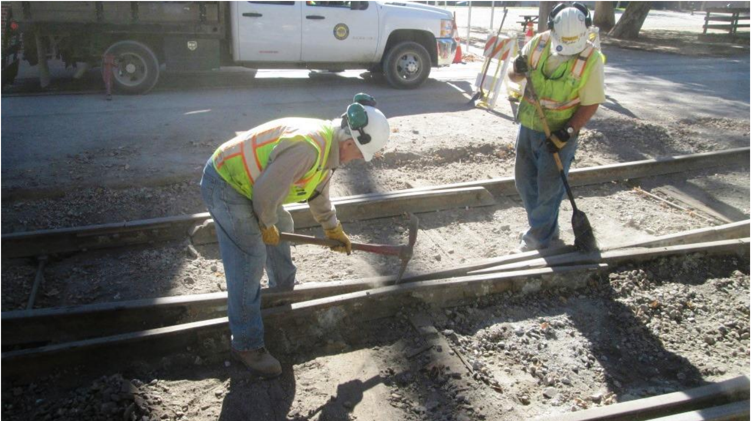
Mike W. breaks-up concrete stuck between the converging rails in the frog while Mike F. clears the flange-way
