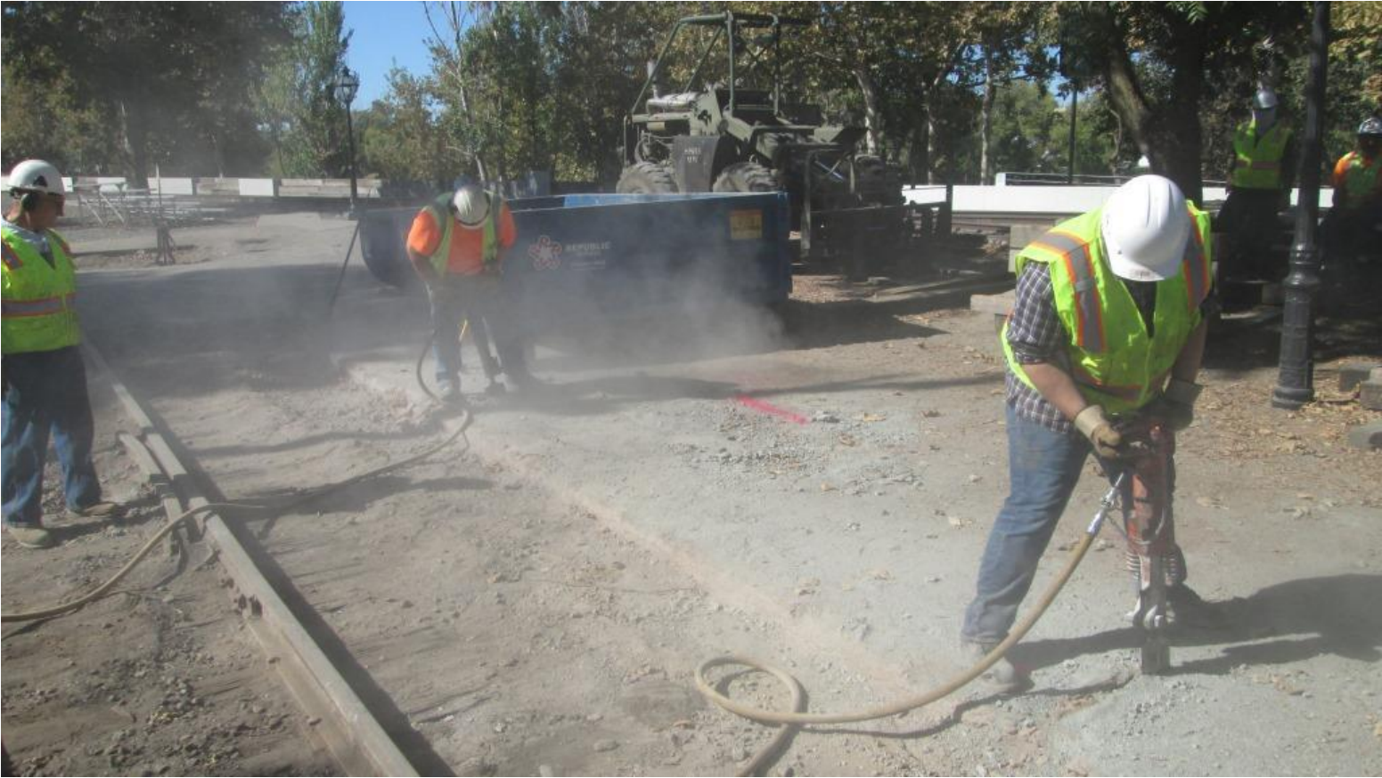
Once again, the jackhammers make an appearance as Frank and Josh begin breaking up the soil-cement
