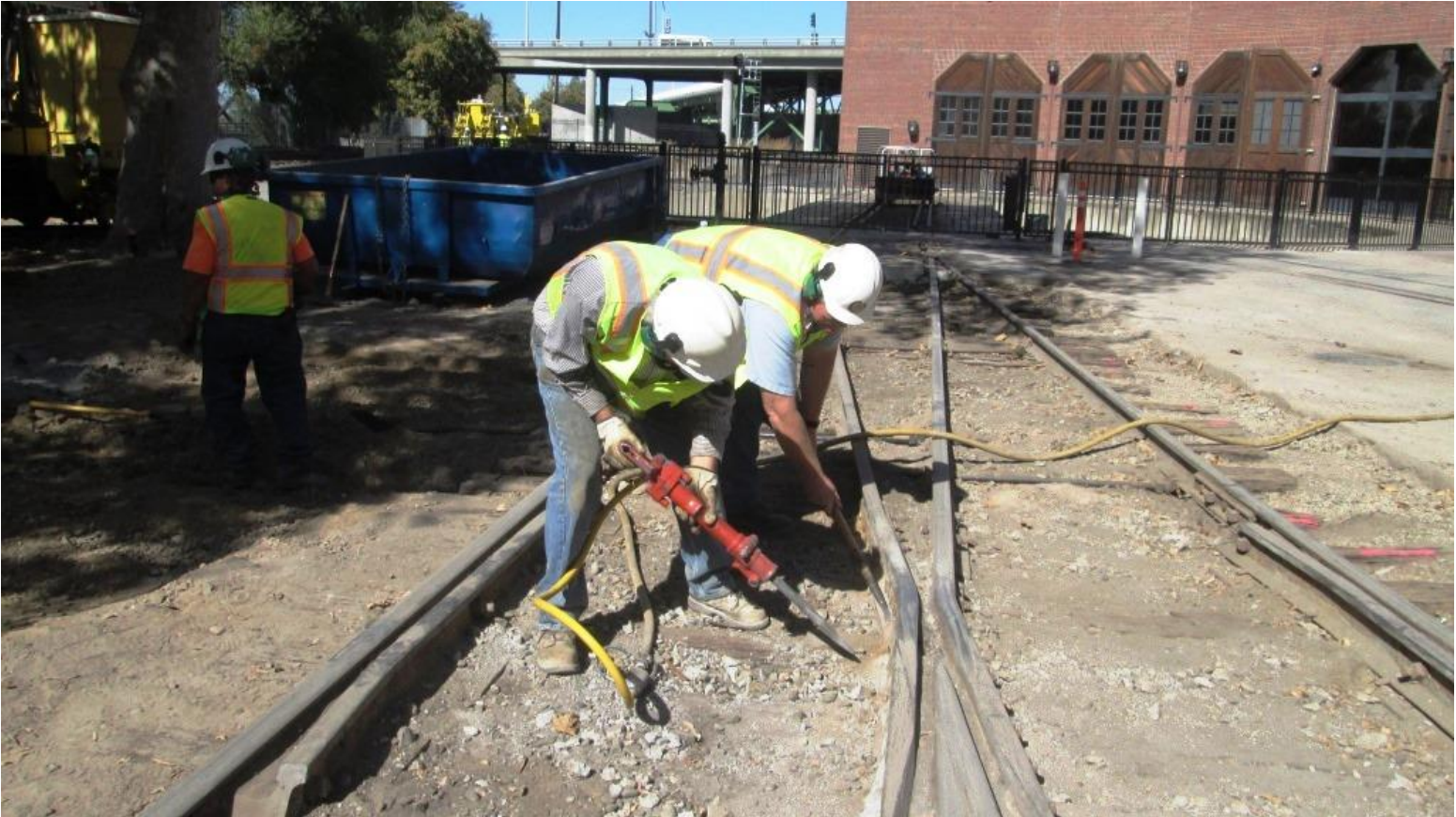
Steve and Chris chip-away at the concrete stuck between the bolts of the frog
