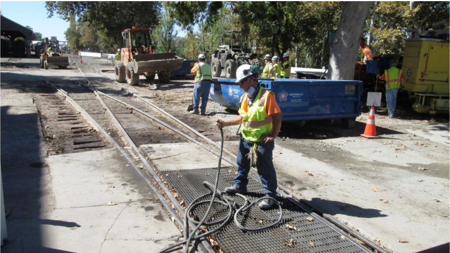
The dust mitigation program came to a quick end due to lack of water pressure
