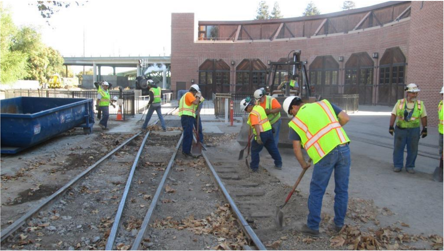
It's Saturday and, having devoured the doughnuts, the Team gets right to work removing debris from on top of the ties
