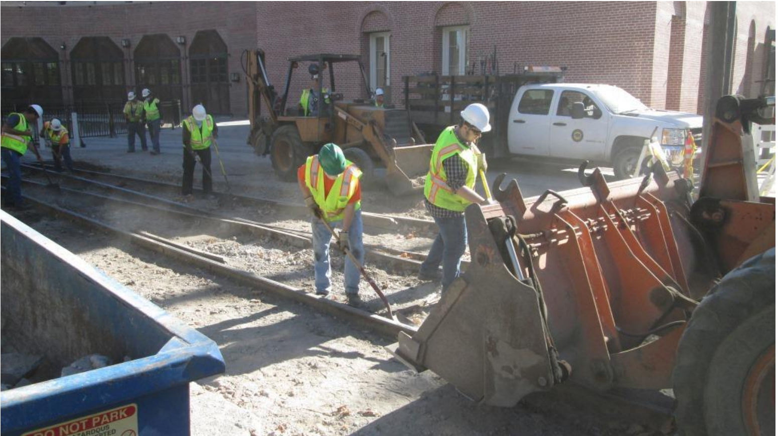
Frank brings the loader in for Tom and Josh to start filling the bucket
