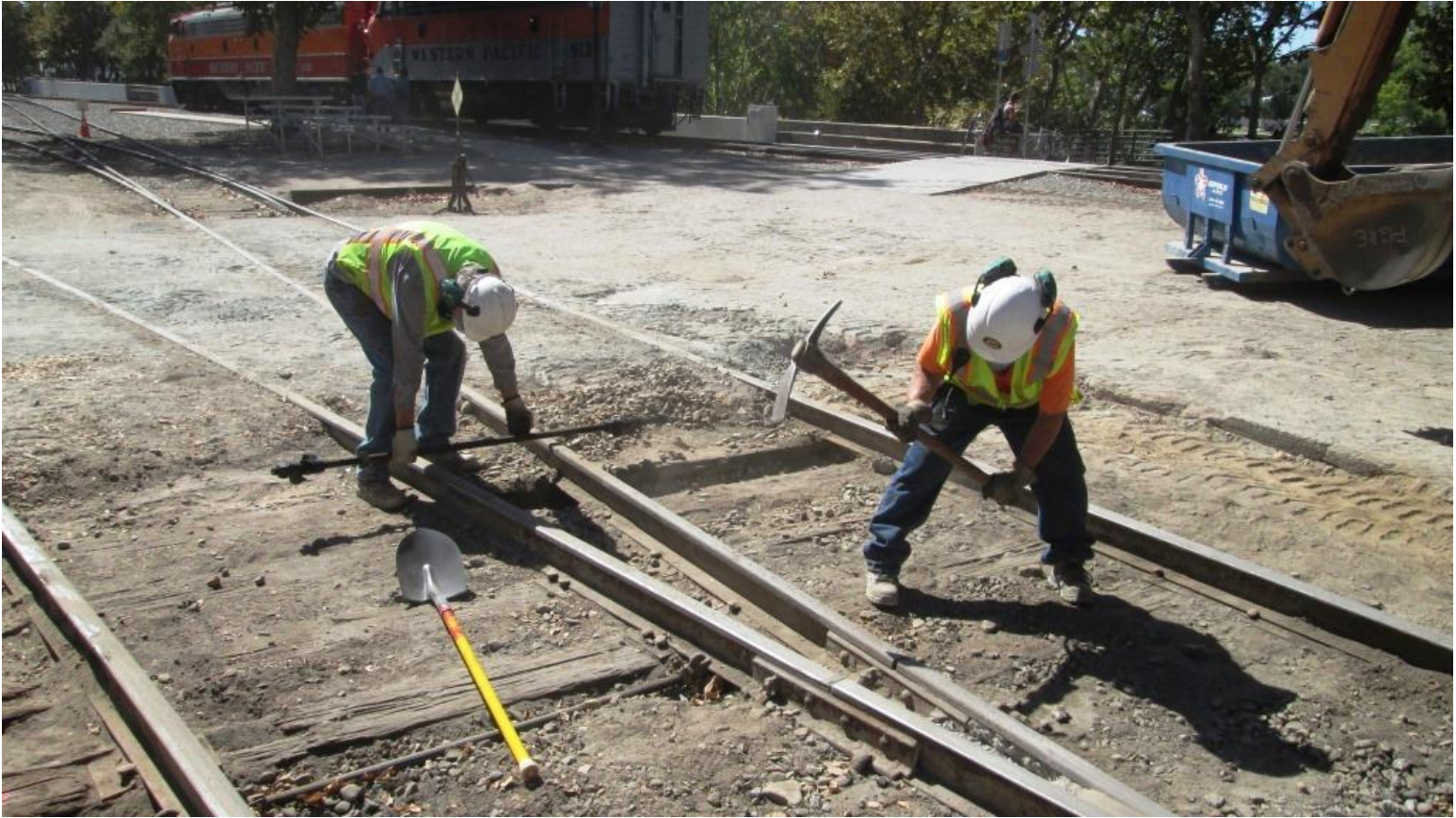
Steve gets a gauge-rod ready to install as Joe digs out a crib for another gauge-rod
