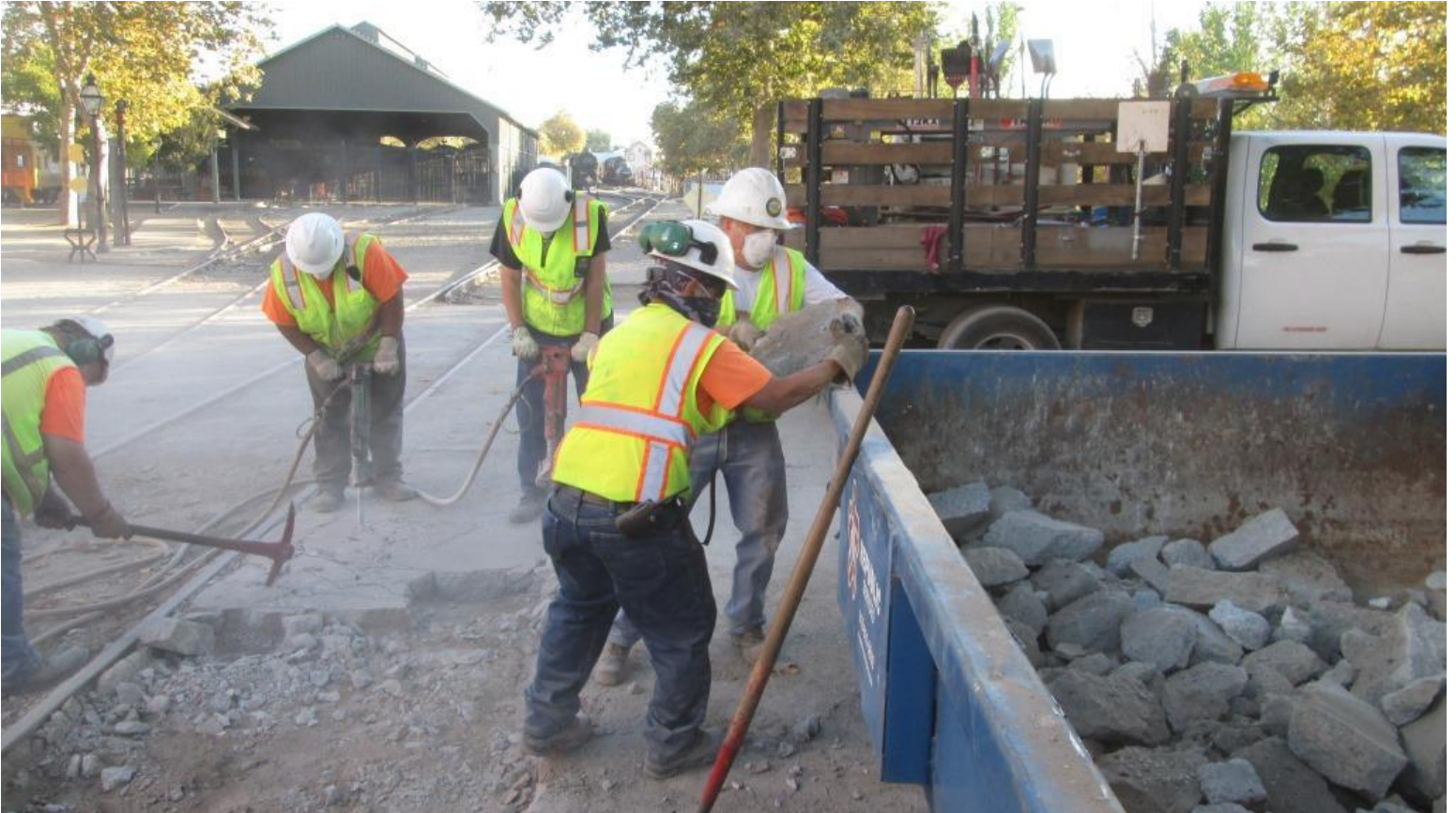
Joe and Mike H. lift a hefty chunk of concrete into the dumpster
