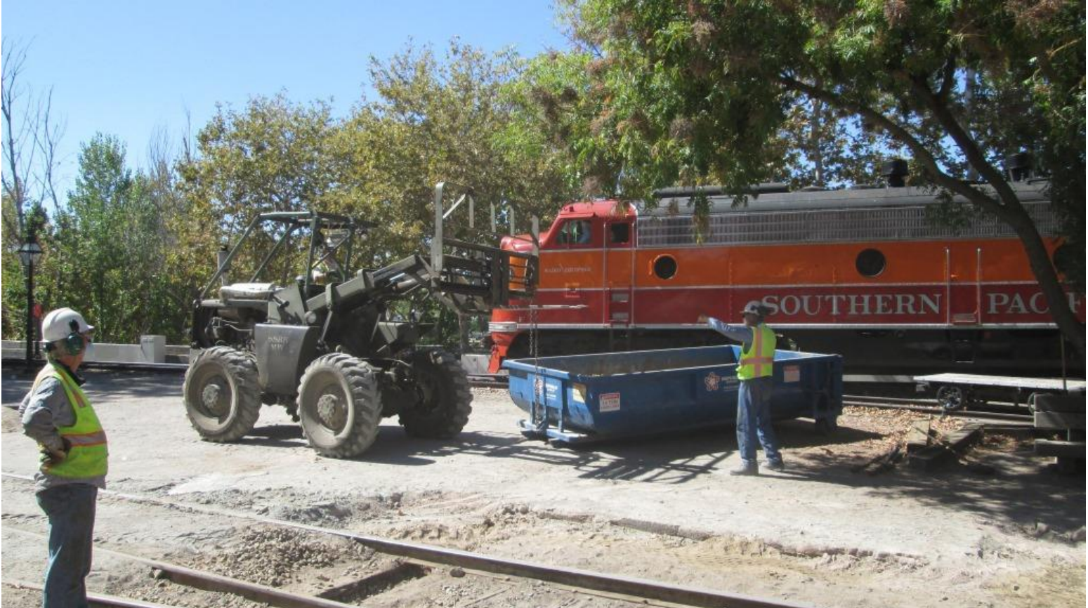
Talk about being alert to train movements, Mike F. and Alan reposition the dumpster as the 6051 passes by on the Old Main
