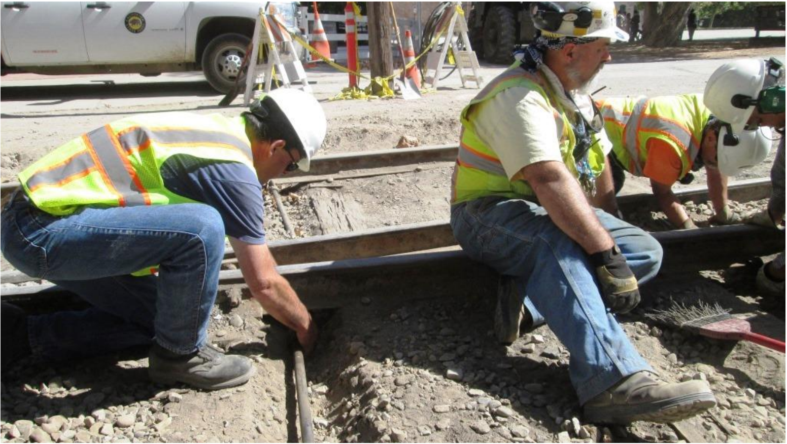
Andrew secures the next gauge-rod on the east rail...
