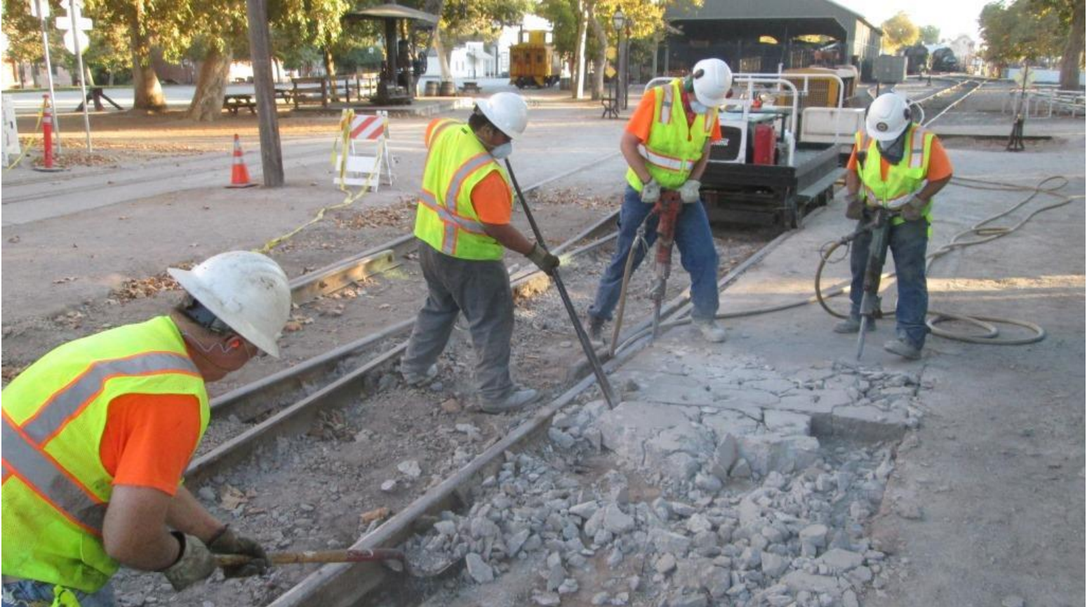
Mike H. and Anthony work the debris loose as Weston and Joe keep the jackhammers going
