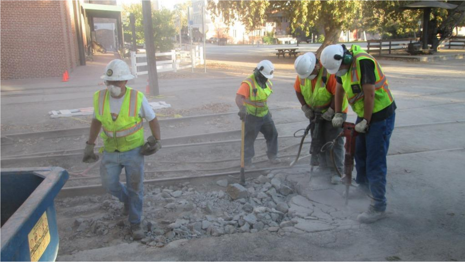
Getting to the end of the line: Anthony and Weston break-up the last bits of concrete
