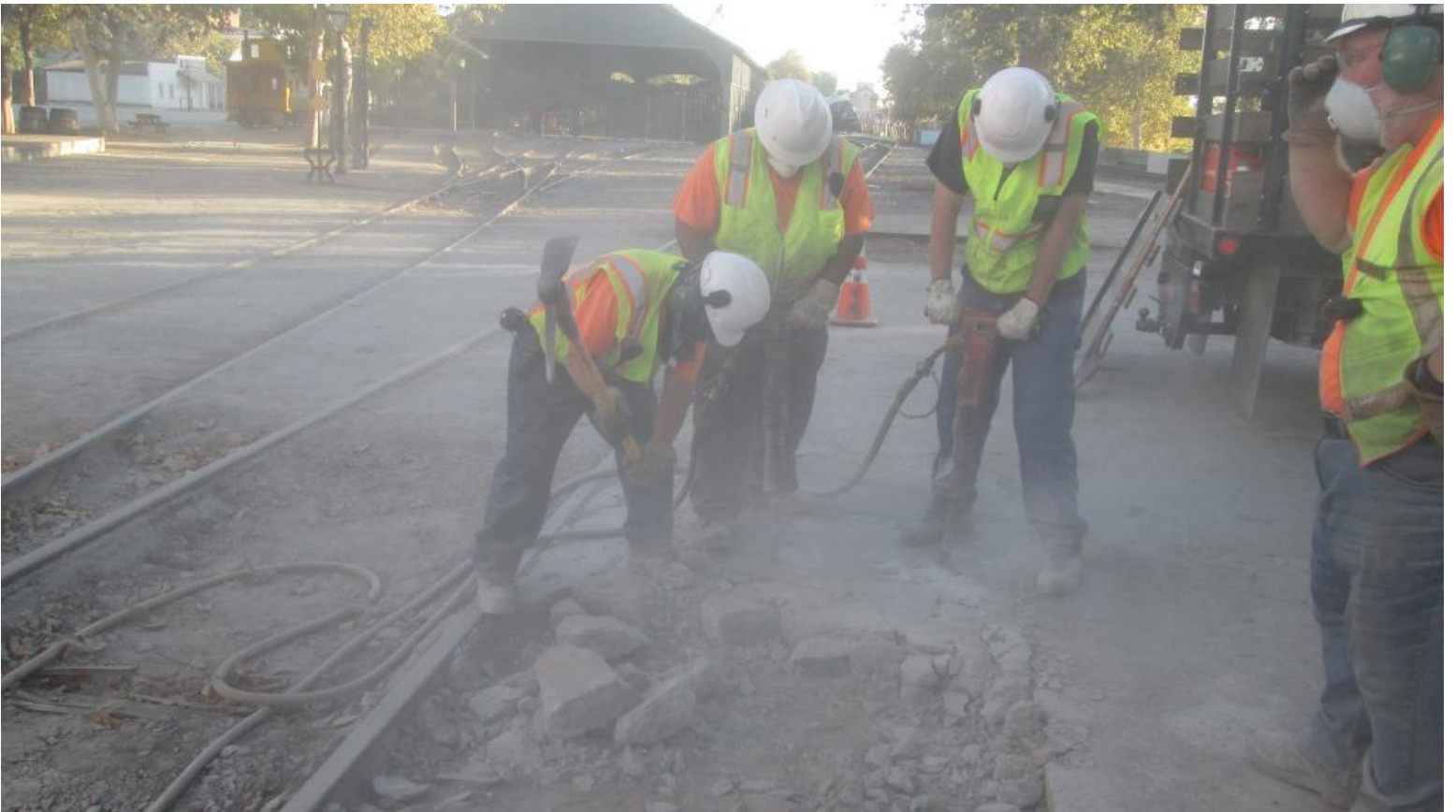
Joe picks loose the chunks for easier removal
