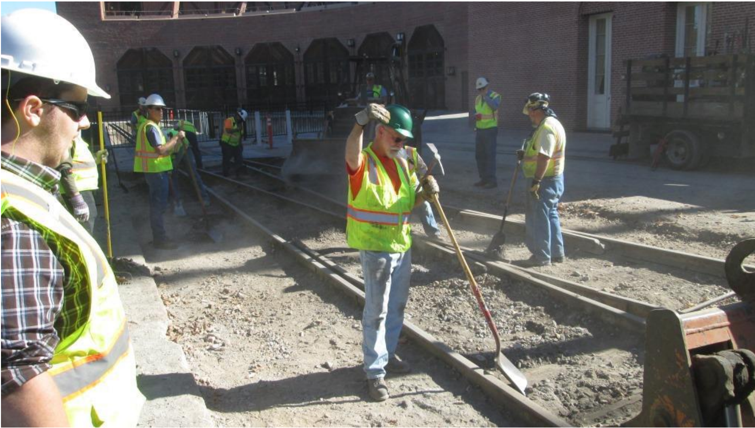
Tom provides direction to Frank in the loader
