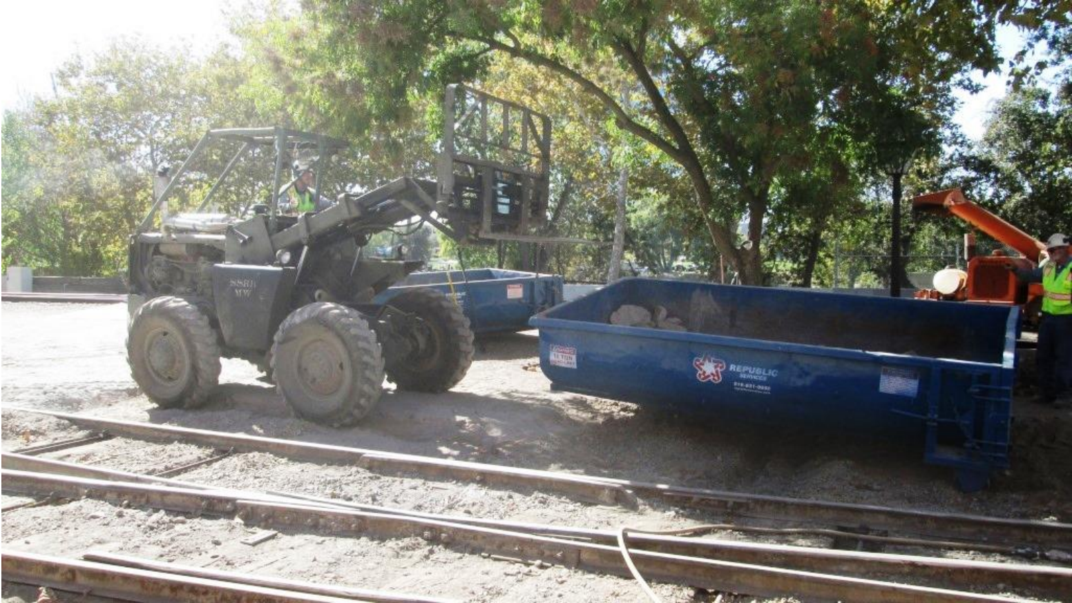
With work winding down, Steve on Big Green, moves the other dumpster into position for pick-up
