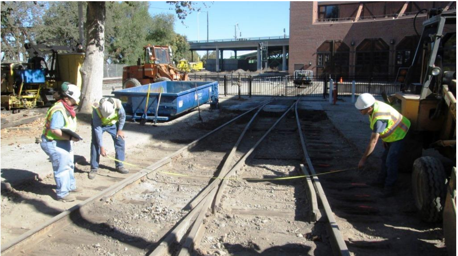
Heather records the findings as Alan and Andrew measure the ties marked for removal
