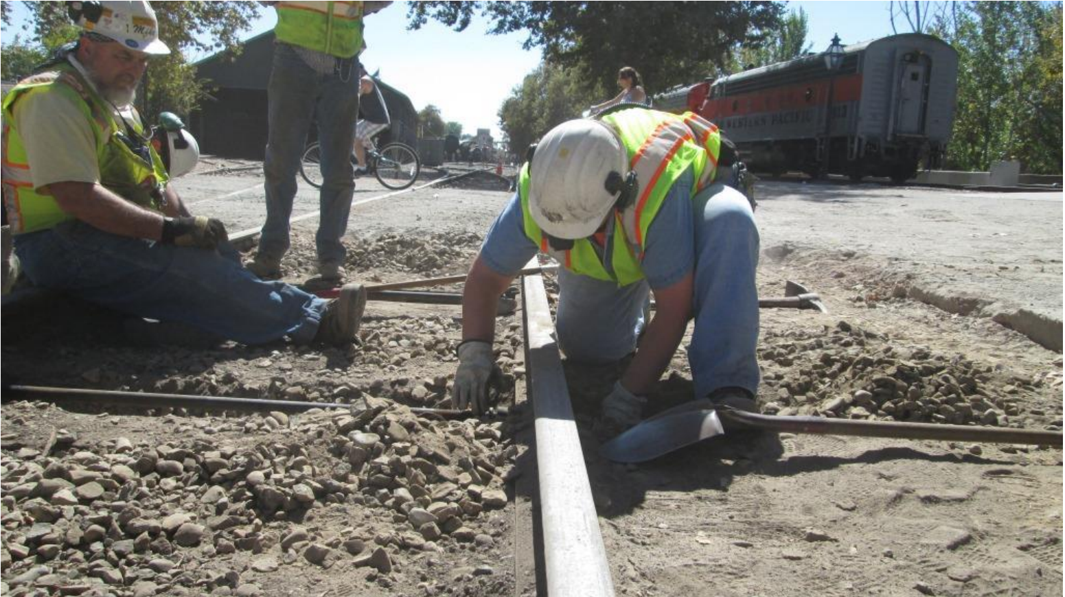
...While Heather secures the clamps onto the west rail
