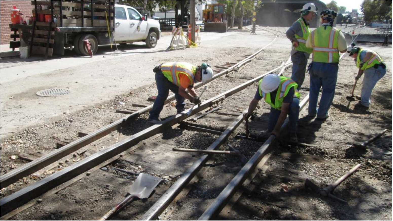
Joe and Andrew get the next gauge-rod installed
