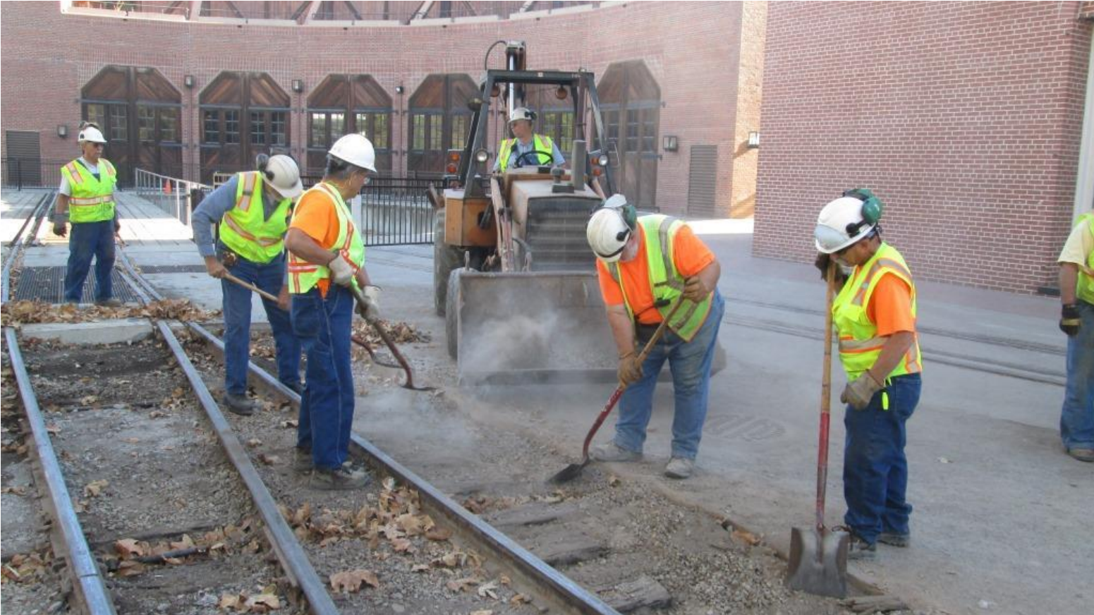
Chris brings in the back-hoe as Alan, John, Frank, and Joe fill the bucket with loose rubble
