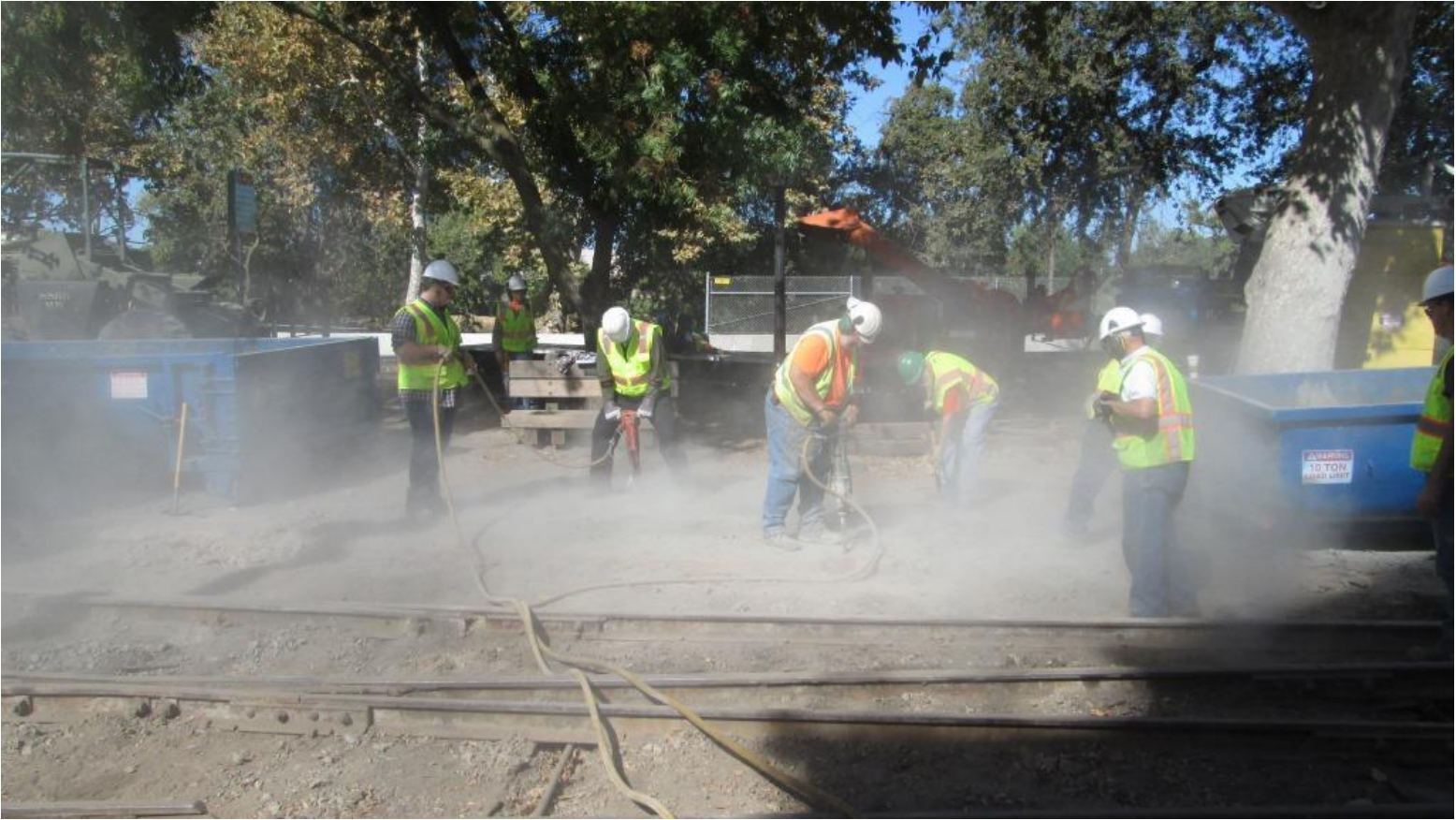
Jose takes a turn with the jackhammer and Josh guides the hose. Frank, Tom, and Clem keep the dust flying
