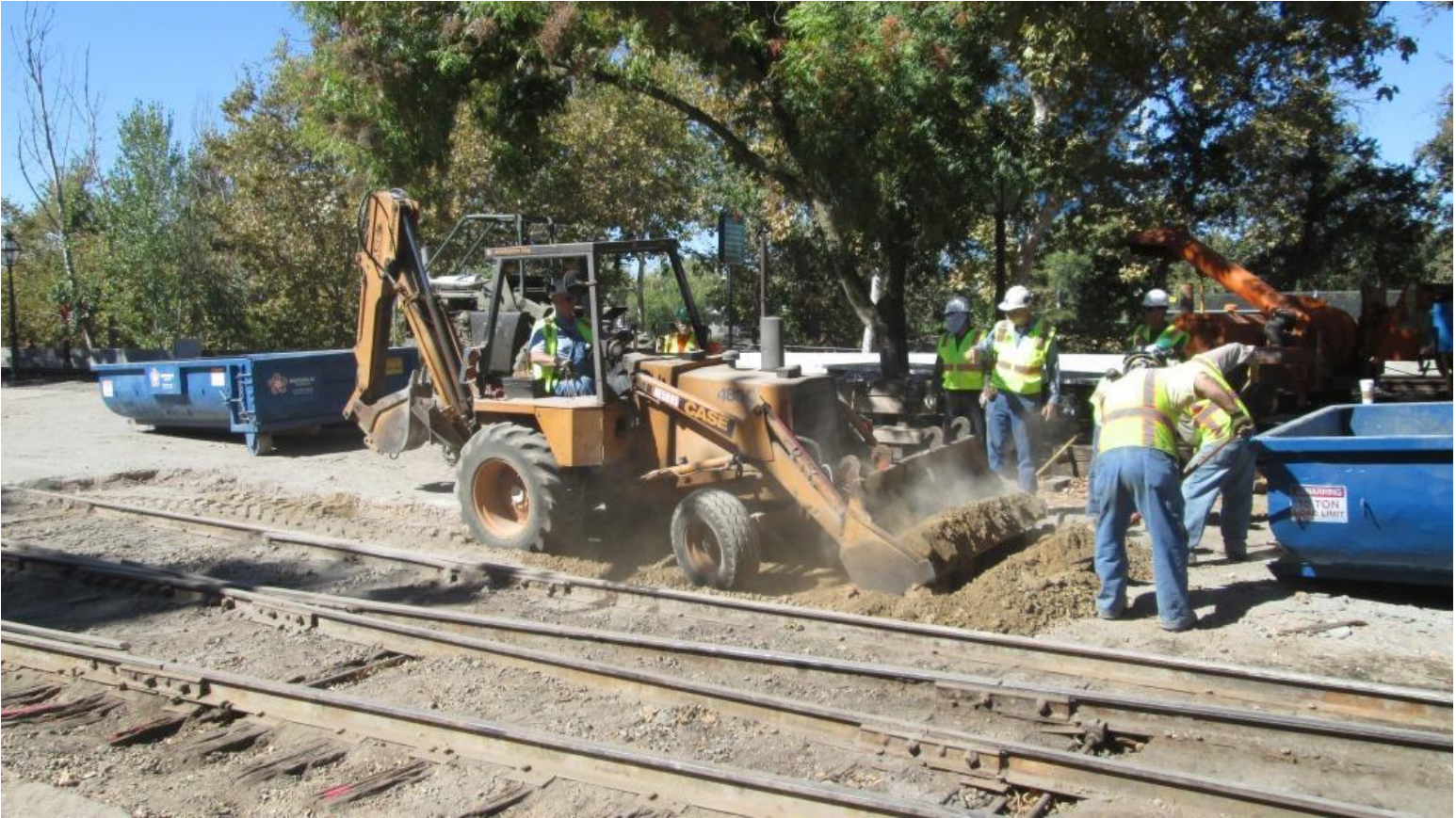
With the soil-cement broken up, Chris started digging with the back-hoe
