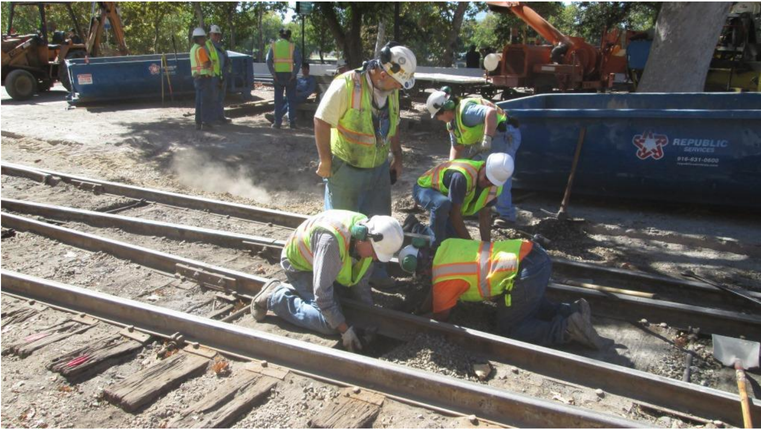
Gauge-rod number three is installed
